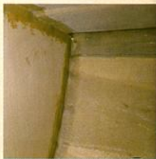
Bulkheads are laminated to deck and with an Airex cushion
